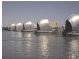
Figure 13: The Thames Barrier.
